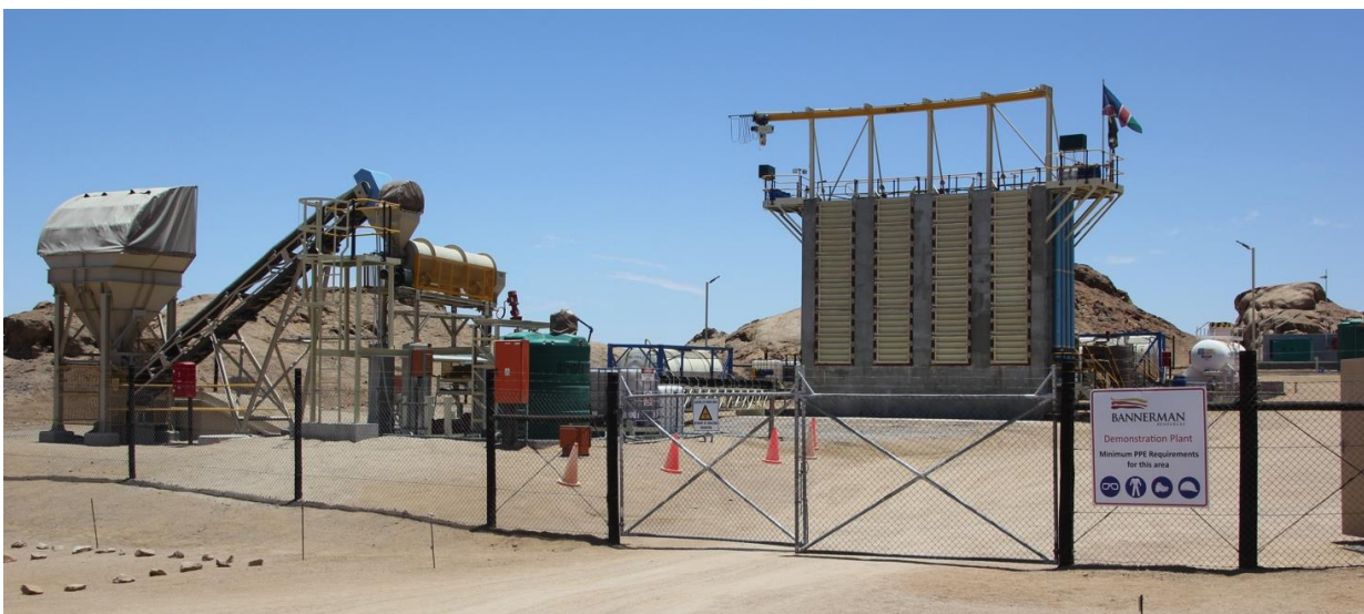
Figure 1 - Etango Heap Leach Demonstration Plant
