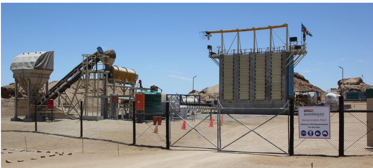
Figure 1 - Etango Heap Leach Demonstration Plant
