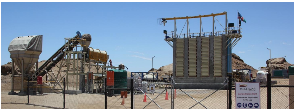
Figure 1 - The Etango Heap Leach Demonstration Plant, above, has provided improved recovery and reagent results that can be incorporated into a revised Definitive Feasibility Study.
